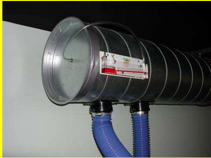
Duct Static Pressure Sensor
